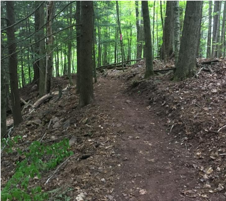
Full Bench Sidehill – 3 feet width
