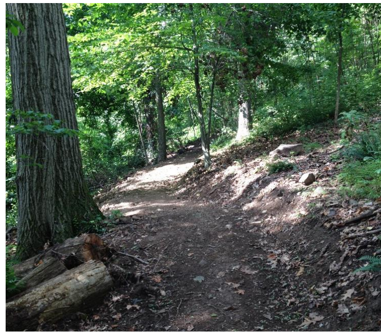
Full Bench Sidehill – 4 feet width
